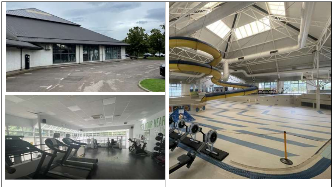
Figure 4.1 – Images of the Current Pool Facility
